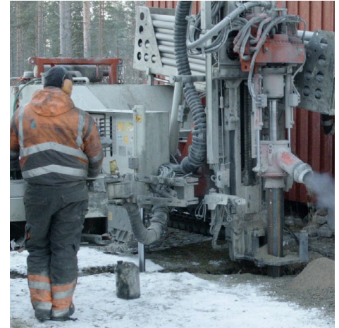
Drilling of a borehole for residential geothermal heating in Northern Finland. Geothermal is an ideal winter heating option because the ground is constantly warm. The rack of tubes is full of drill extenders. Well depths for Massachusetts measure in the hundreds of feet. Public Domain Olli Niemitalo
