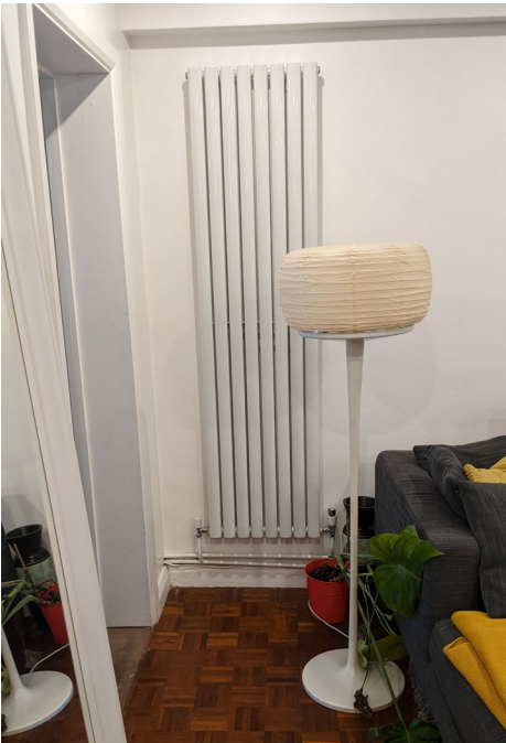
U.K.-style panel radiators are unlike anything we have in the U.S. This seven-foot tall panel radiator radiatively and convectively heats a 300 square foot living room, and wilts a houseplant placed unfortunately close to it. CC BY-SA 4.0 MassLandlords, Inc.
