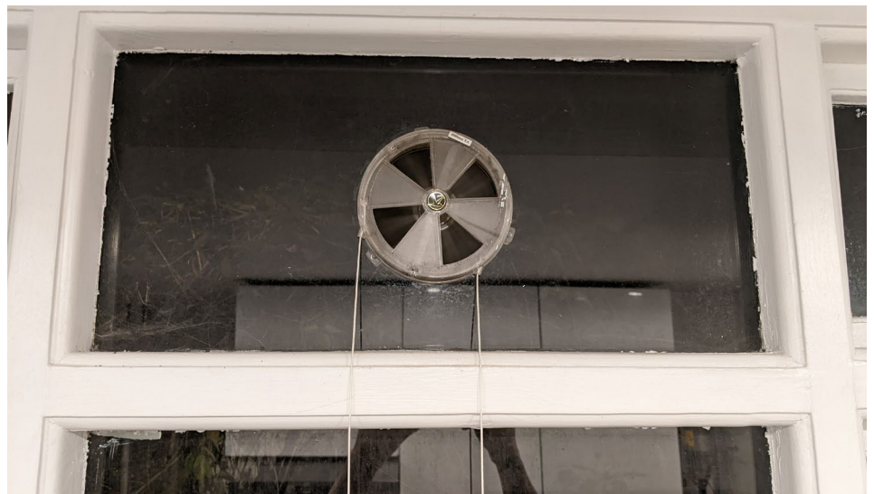
This U.K. window vent is a plastic circle cut into the glass pane with six fins. The fins can be closed by pulling on the string. In colder climates like Massachusetts, we wouldn't dream of doing this. CC BY-SA 4.0 MassLandlords, Inc.
