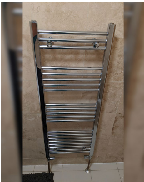
Hot water runs through this UK-style towel rail and bathroom heater. The bathroom stays warm. Towels stay hygienically dry. CC BY-SA 4.0 MassLandlords, Inc.
