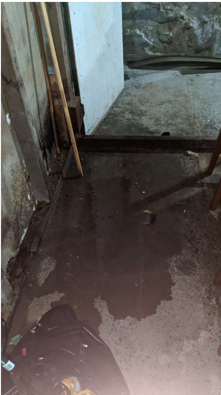
When shopping for an unoccupied property, a wet basement clearly means a problem with the building. This basement was soaked because the first-floor renters were not using a shower curtain. (Lic: CC BY-SA MassLandlords, Inc.)
