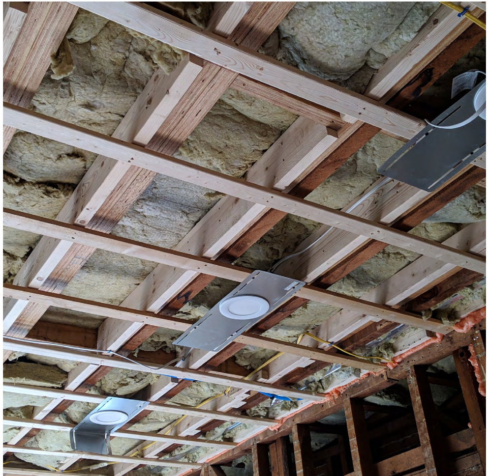
Rock wool (yellow) is visible stuffed between the joists of the floor above. The bays do not need to be full, as in insulation. There should be an air pocket above and below the rock wool to reduce noise travel. CC BY-SA MassLandlords
