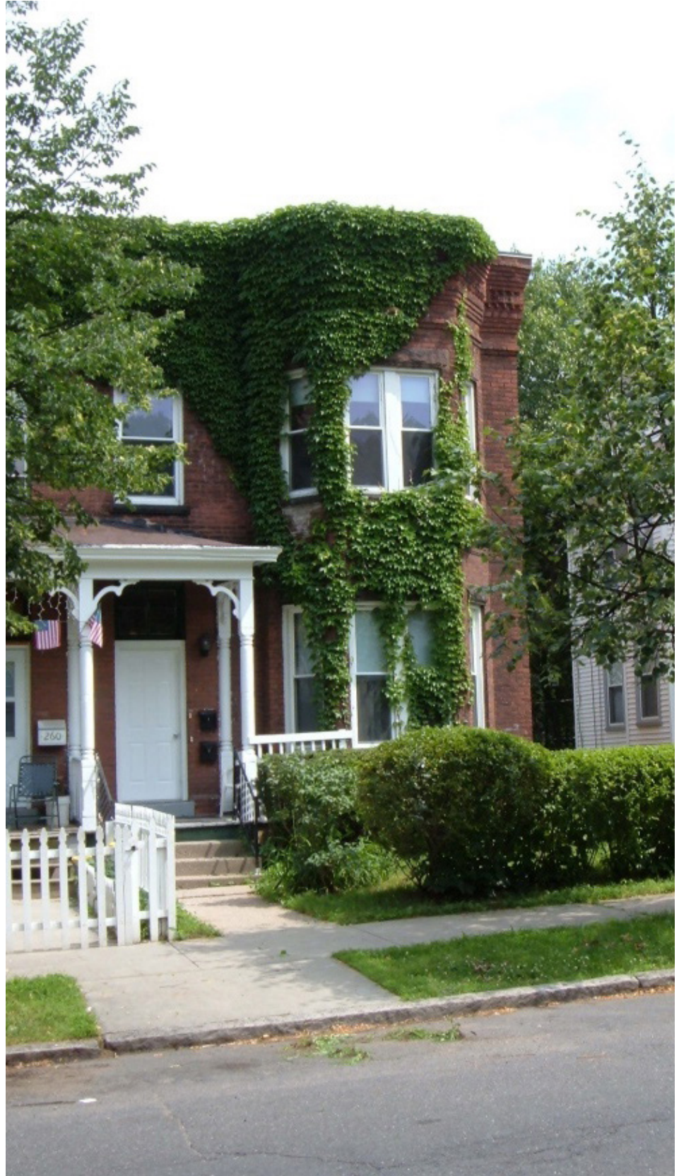
Jo Landers invests a lot of sweat (and blood) equity in her rental properties, including this historic Holyoke multifamily, where she completed many interior renovations herself. Image: cc by-sa jo landers
