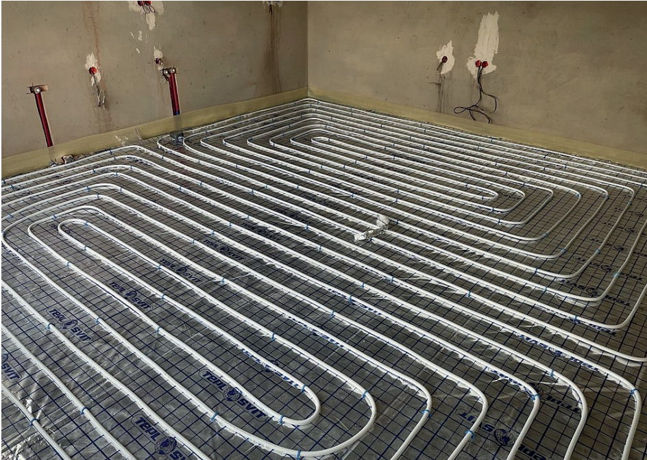
Hydronic radiant floor heating systems install a grid of refrigeration pipes as a sublayer before installing flooring over the pipes. While these systems can be expensive to install, they are the most efficient hydronic systems available and provide high quality heating. Image: cc by-sa Wikimedia commons-Viii23dawari.
