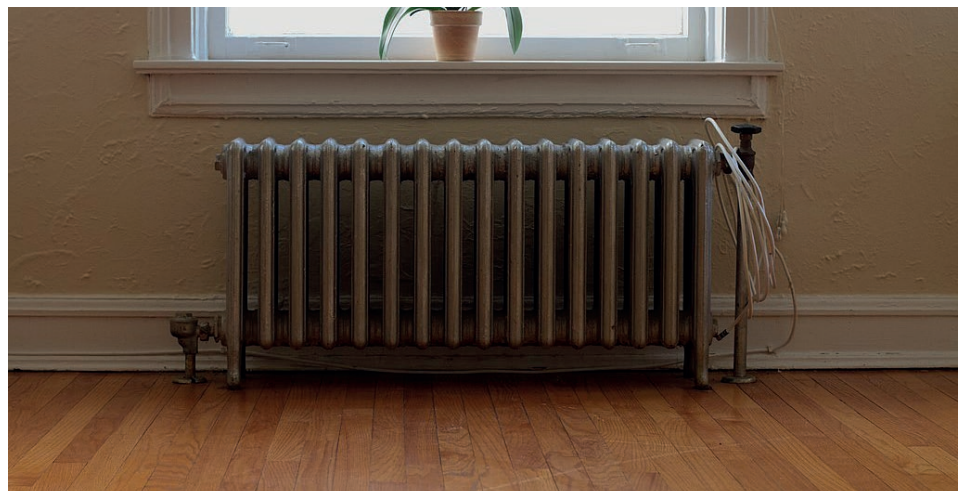
Steel radiators like this one are a ubiquitous sight in triple-deckers and multi-families built in 19th and 20th centuries. Designed to last, these hydronic systems are still effective for providing heat – in some cases, too much heat. Image: cc by-sa Wikimedia commons.
