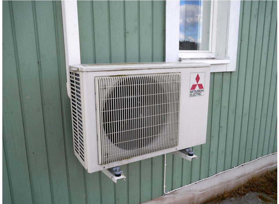
Converting to a non-fossil fuel-based system like a heat pump can be expensive. However, incoming federal dollars may help many residents with the cost. (Image: cc-by-sa Santeri Viinamaki)
