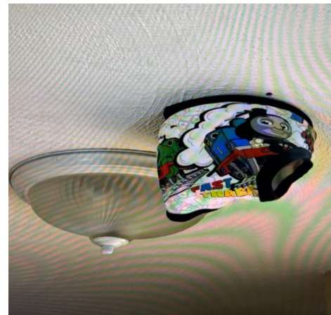
This real image from a Massachusetts apartment shows what one renter did to prevent smoke setting off their alarm. This would be hilarious if it weren't potentially deadly. CC BY-SA 4.0 MassLandlords
