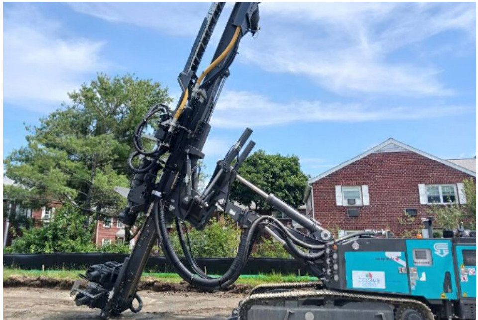
Eversource, one of the state's largest gas companies, bored 90 holes deep into the neighborhoods around Concord Street in Framingham to create a series of pipes as part of its geothermal network pilot. The state's new climate law allows gas companies to broaden their scope of service to add geothermal energy service. Image: Eversource source photo.
