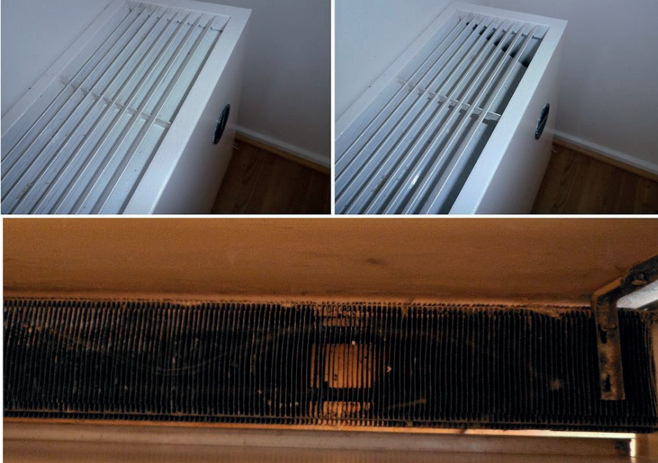
Forced hot water baseboards like this unit produce high-quality, consistent heat by radiating warm air through a tightly aligned series of aluminum fins, as shown in the bottom frame. The top two frames show the baseboard radiator's cover with top vent closed and open. A drop-in air-to-water heat pump would allow owners of these types of systems to keep them in place in their homes and rentals. Image: cc by-sa Tomakkermans Wikimedia commons
