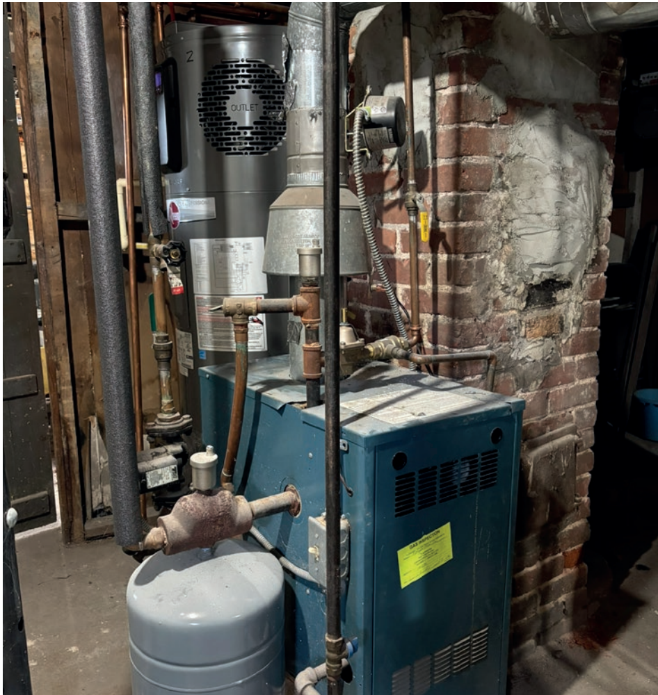
This old boiler (blue) is similar to many that are ideal candidates for air-to-water heat pump replacement. The copper forced hot water lines are at left of frame and insulated. The boiler, gas line (center of frame) and combustion exhaust can all be removed. A refrigerant line set can be run from this location to an exterior condenser a few feet away. The heat pump can be placed where the boiler and exhaust once stood. There would be no need to enter any of the rental units above. In the background, a heat pump water heater stands in the place of a gas water heater. CC BY-SA 4.0 MassLandlords
