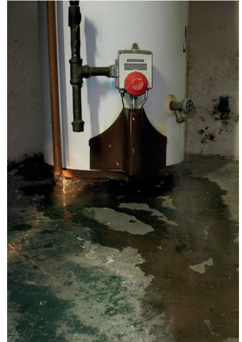
If you notice liquid running or leaking from your water heater, like this one, it's probably time to replace it with a heat pump water heater. Cc by-sa flickr Rob Ireton
