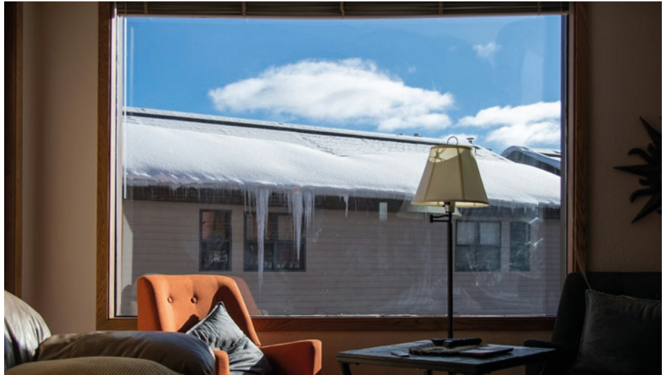
No snow on the roof peak? It could just be a drift, but this is often a sign of heat loss, which can lead to ice dams. (Image License: Nader Saremi for Unsplash)
