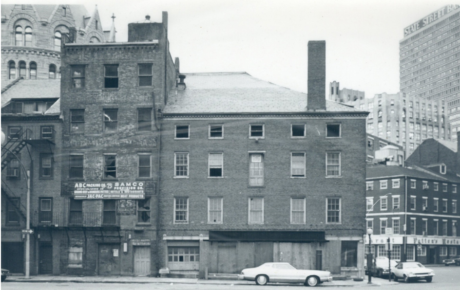
The Jenney building on Central Street, Boston, pictured here circa 1970s-'80s, with its boarded up windows and street level storefronts, offered an all-too-typical example of urban blight as the city maintained rent control for more than two decades. Will Massachusetts voters elect to return to this by approving rent control mandates on the November ballot? Image: CC BY-SA flickr-City of Boston copyright.
